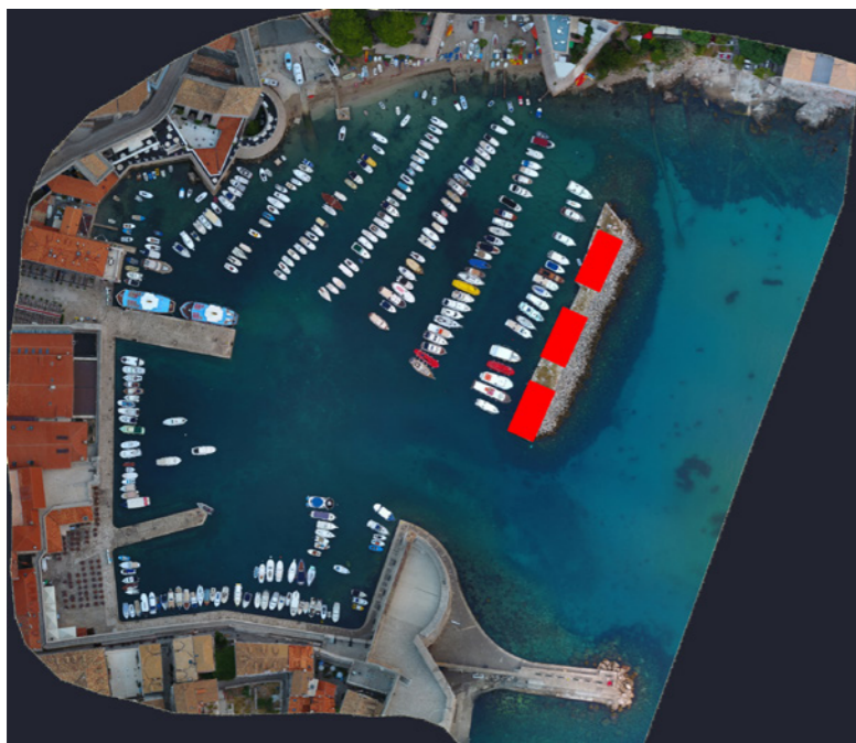
Fig. 29a-d Building phases of the Kaše breakwater, according to recent discoveries: a) Tripartite breakwater built from 1484 to 1487 (represented by Konrad von Grünenberg in 1487); b) Three parts connected in 1498 and 1501 (represented by Nikola Božidarević, around 1500); c) Breakwater extended towards Ploče in 1514 (attested by the archaeological survey); d) Breakwater reconstructed after the destruction of its northern part, certainly before 1618 (present-day situation), (I. Radić Rossi)
